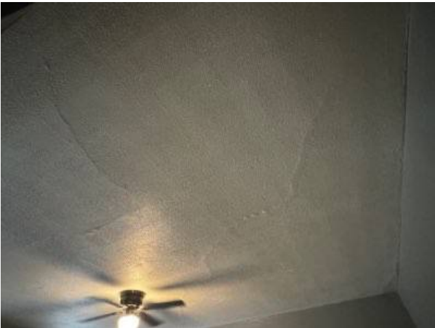
Photo 22-1 Dining room ceiling
