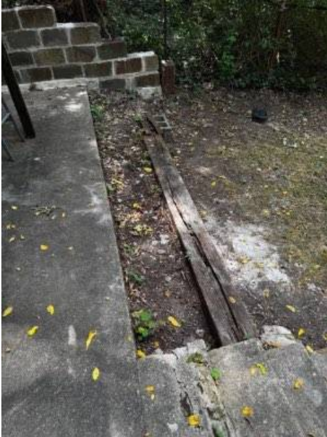
Photo 2-1 backyard retaining wall
