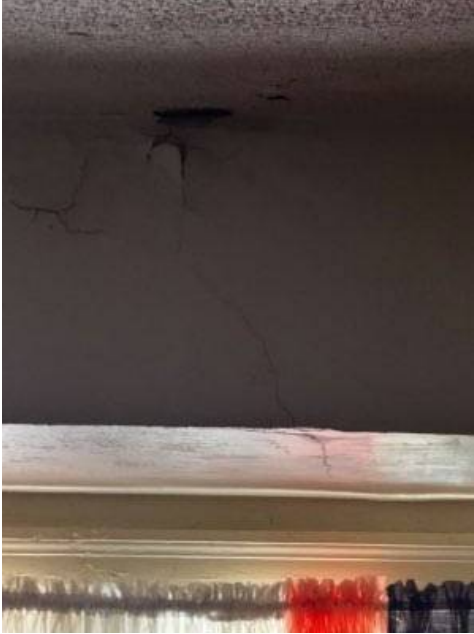
Photo 11-1 roof was replaced in 2024
