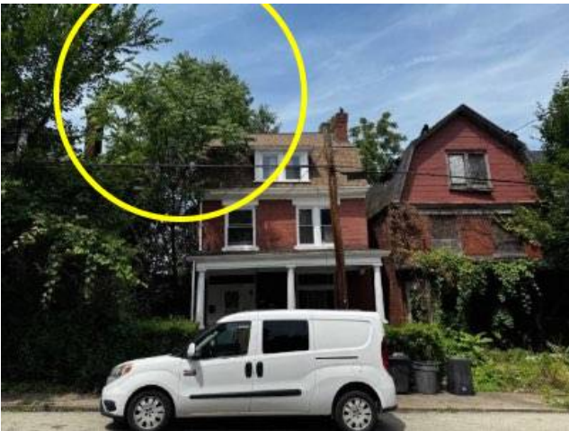
Photo 5-1 Tree touching left side of house
