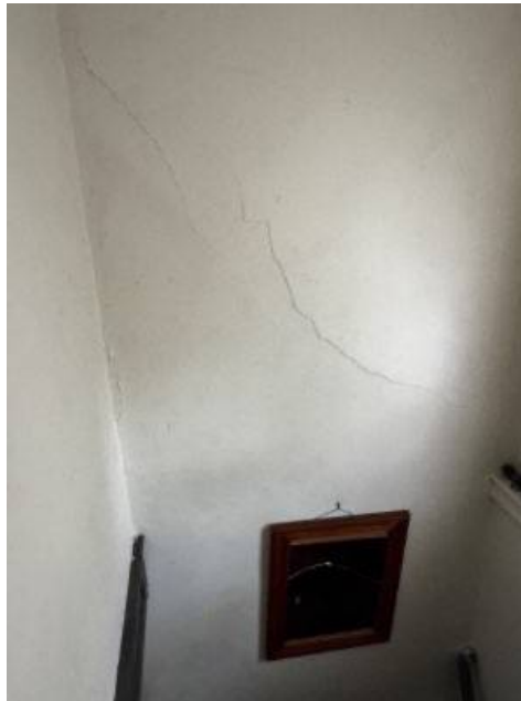
Photo 22-2 Living room ceiling
